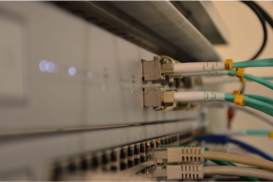
Transceivers are commonly utilized in servers, as seen above, to transmit and receive fiber optic signals.
